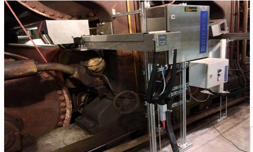
Nonwoven felt fabric installation
