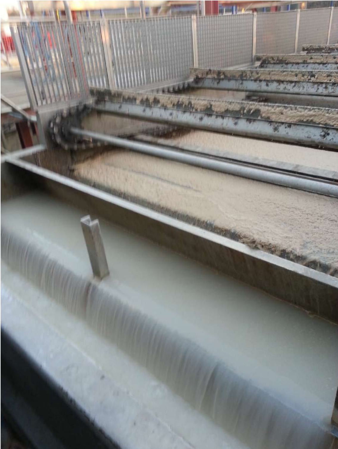
Picture 1 : First stage of flotation before to begin the changes of the existant equipment ( water presurization with air to create micro-bubbles that float solides and emulsions). Aplication of coagulant / antiemulsionant to brake the lactic emulsions and remove fat of the inlet flow, and after join up in the final stage of flocculation.
